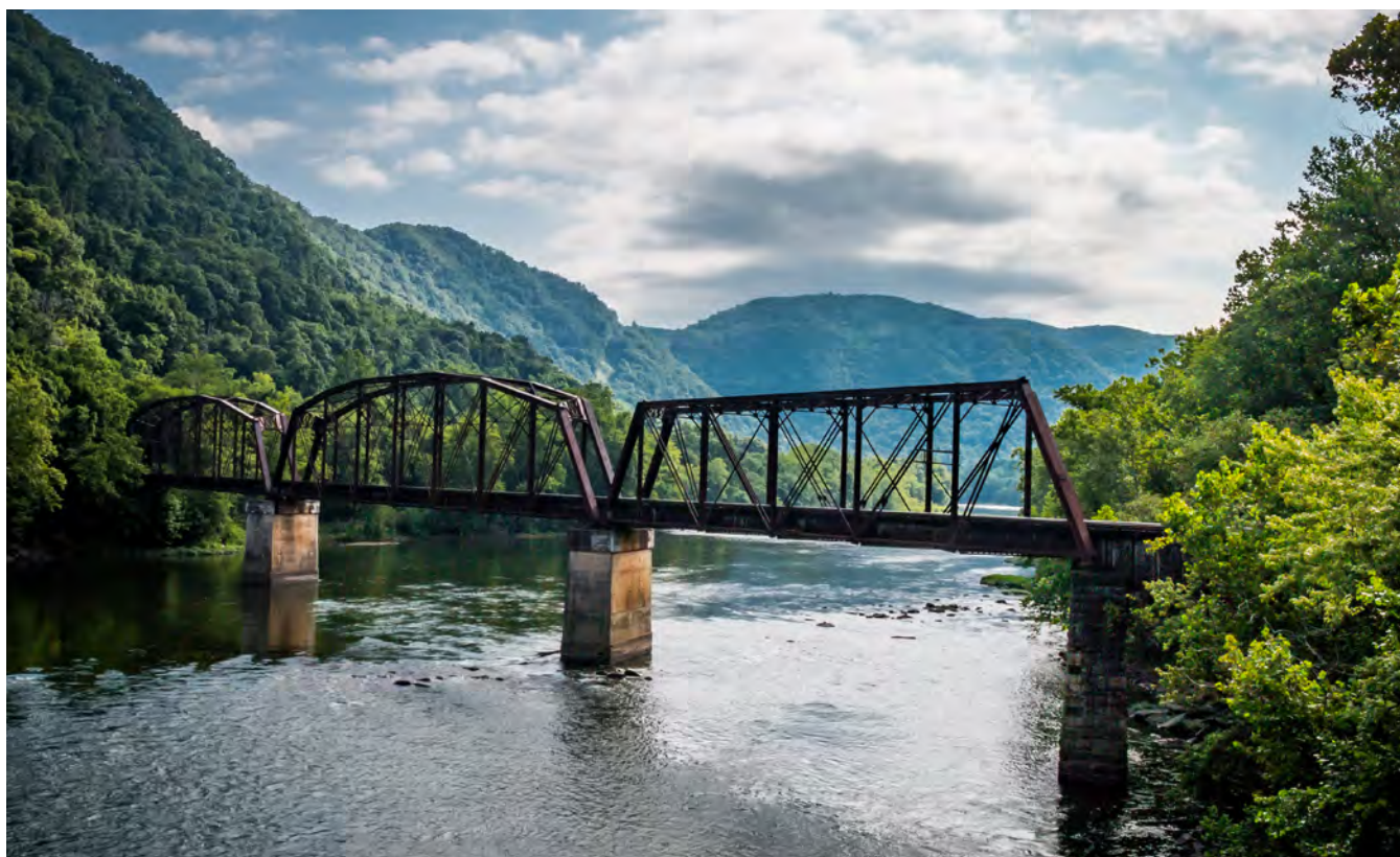
West Virginia Railroad Bridge
